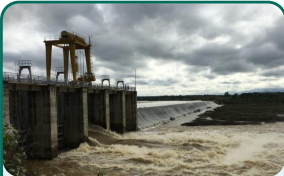
Small hydro, Central Vietnam
